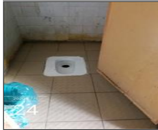
Photo of the sanitary facilities Toilet.jpg
